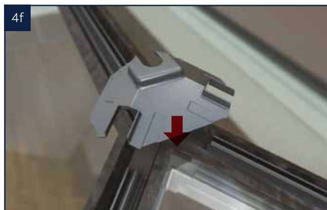
Position the ridge end seal in place ensuring it is central to the hip bars and ridge.
